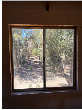
Attic Window noted -Aluminum Frame-
