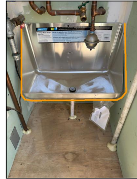
Tankless Drain Pan noted no defects
