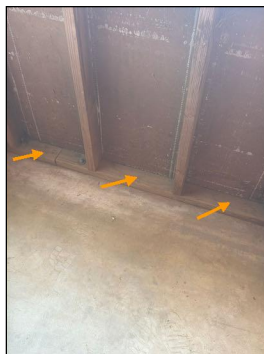
Wall bottom plate no visible defects
