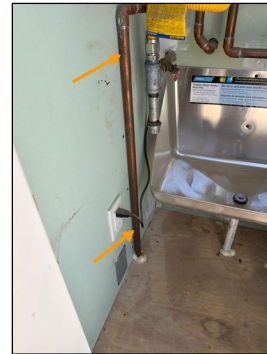
Drain extension pipe no visible defects observed
