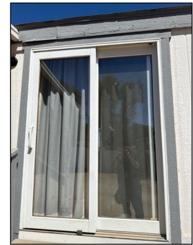
Door 3- Back Living Room Sliding
