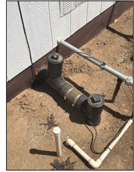
Waste clean out no defects
