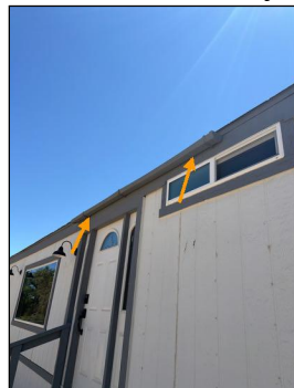
Section of gutter over main entry no defects observed
