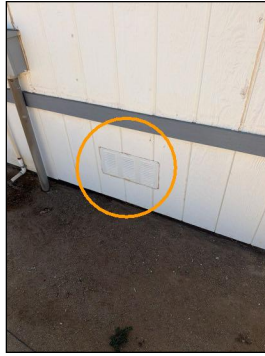
Crawlspace vents located around the perimeter of the home
