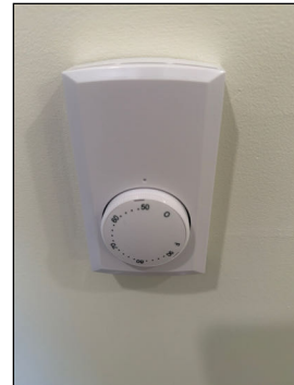
Heater Control in each bathroom
